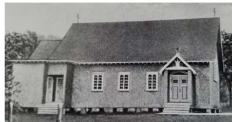
St. Helena Chapel (After Construction- ca 1926)
