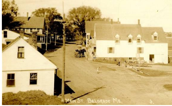
The Taylor Store is the first building located on the right of this picture of the Belgrade Depot. It was demolished in the spring of 2016.
