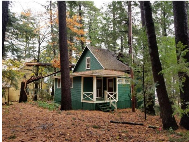
Picture of storm damage above courtesy of Mike Heino
