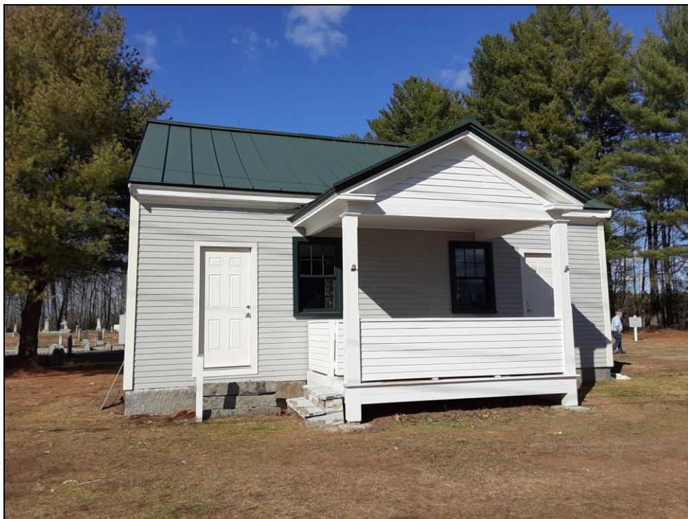
Old Town Meeting House in early May is ready for its final two coats of white paint! [Photo Credit: Dianne Dowd]
