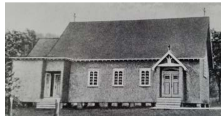
St. Helena Chapel (After Construction- ca 1926)
