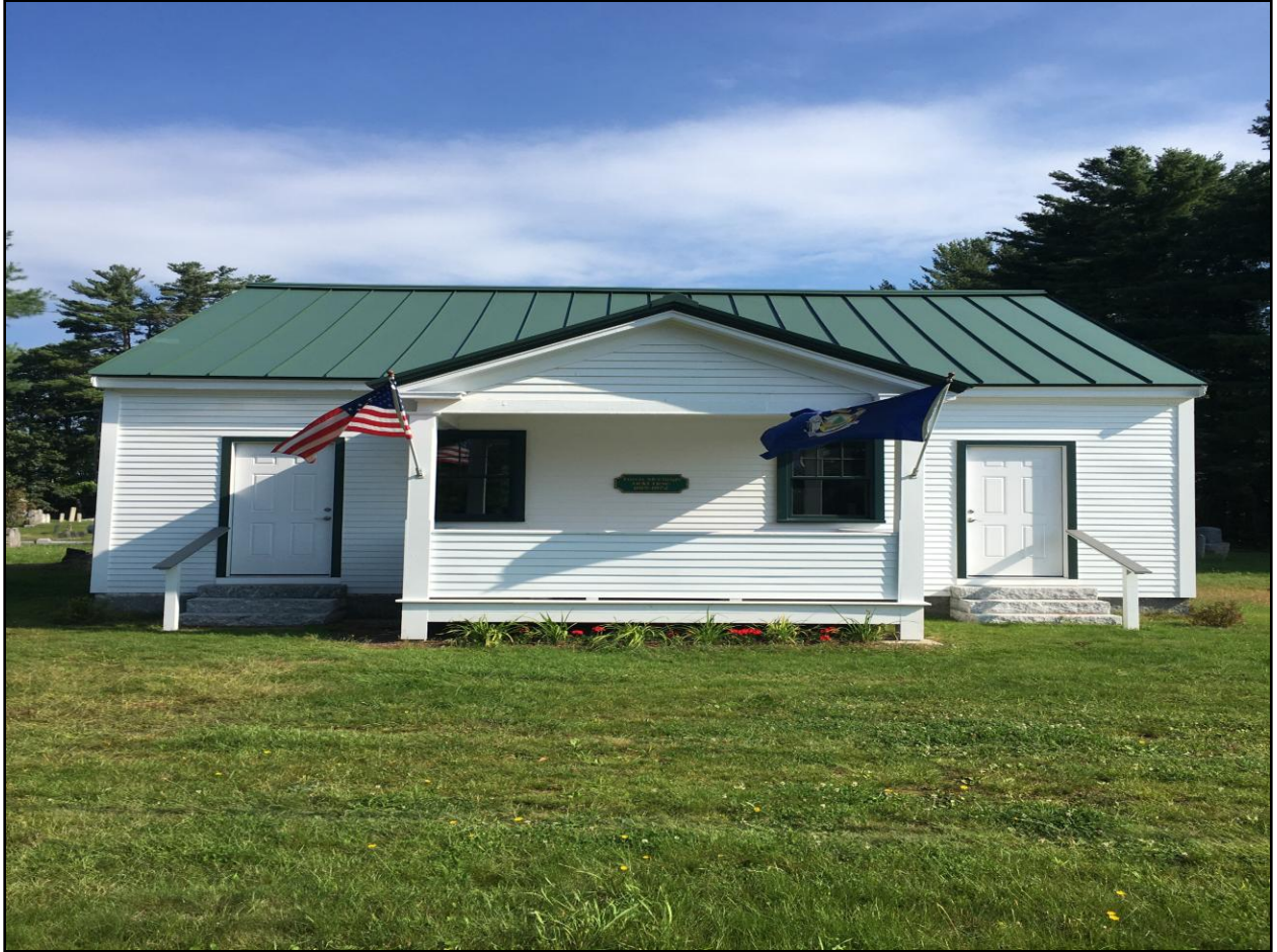
Front view of Renovated Old Town House, with doors, granite steps and wooden railings (Photo courtesy of Rod Johnson)
