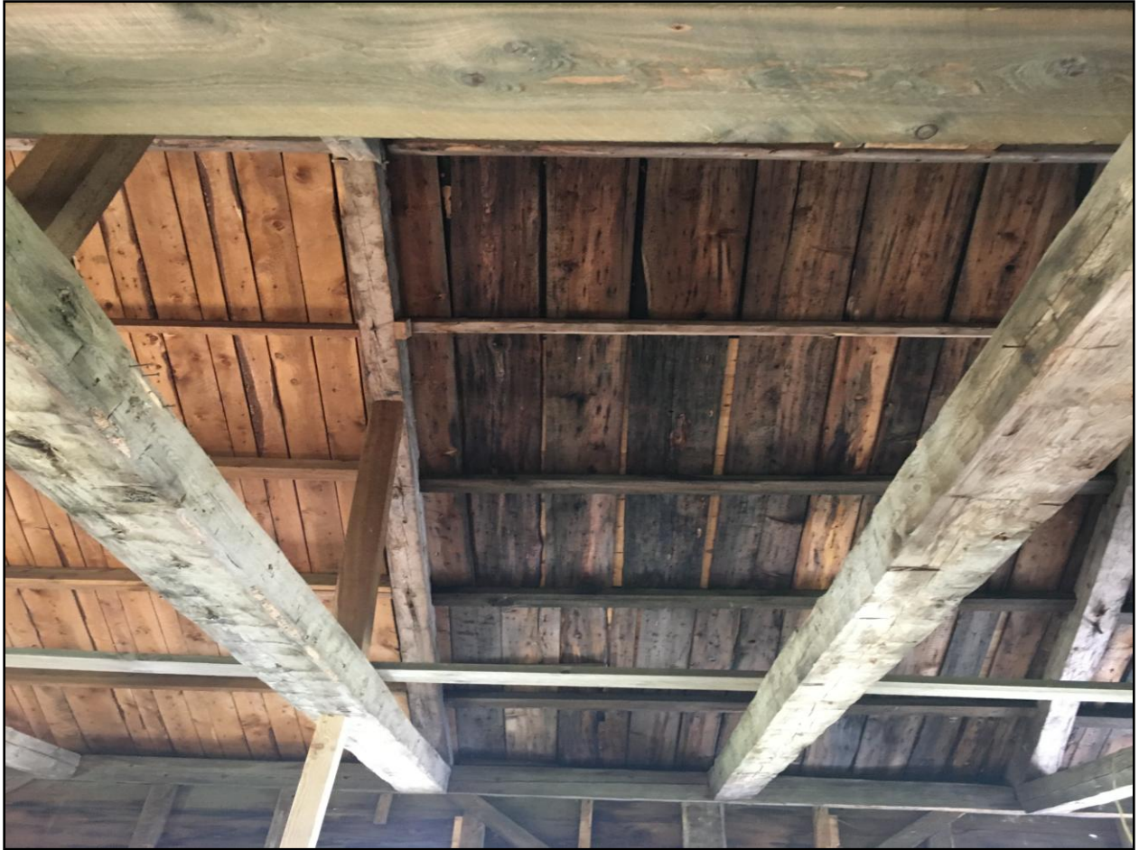
Looking up at ceiling beams with crossties (Photo courtesy of Rod Johnson)
